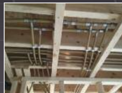
Example of an installation in Monasterevin, Co Kildare. Saving on labour time is 50% over multilayer.
