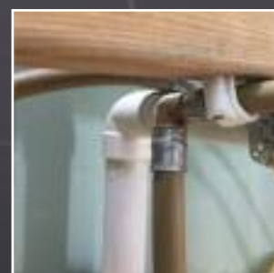
Example of an installation in Kinsale, Co. Cork. Saving on labour time is 60% over compression.
