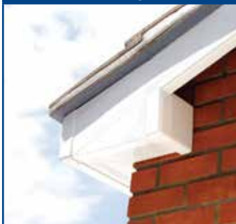
Box End Detail 5: Bargeboard extending to meet the fascia.
